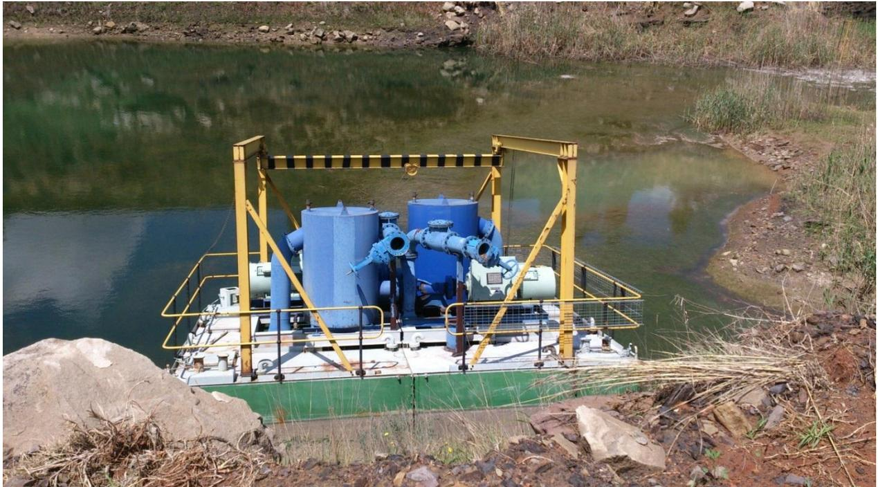
**Figure 4: Extra Barge Mounted Pumping Station**
