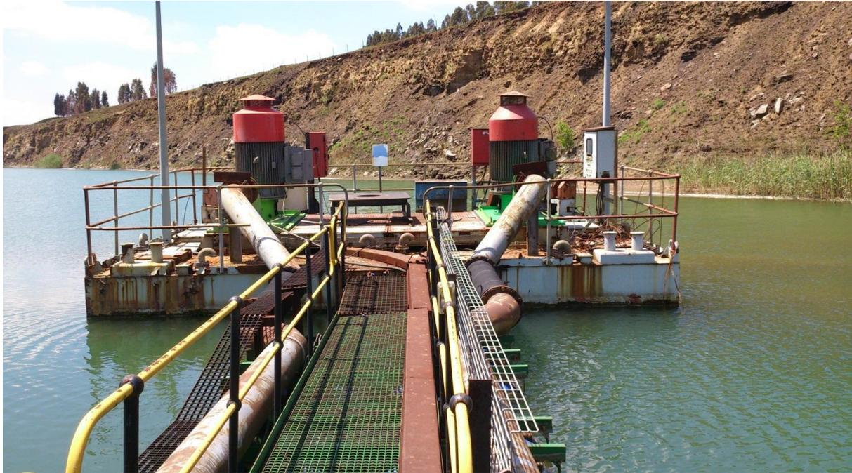
**Figure 3-2: MPS Barge mounted pumping station**
