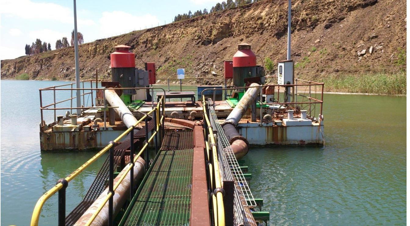
**Figure 2: Matla P. S. Barge mounted Pumping Station**
